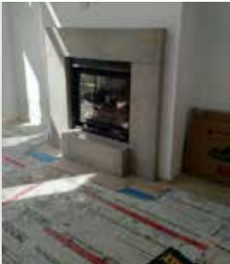
Fire place surrounds
